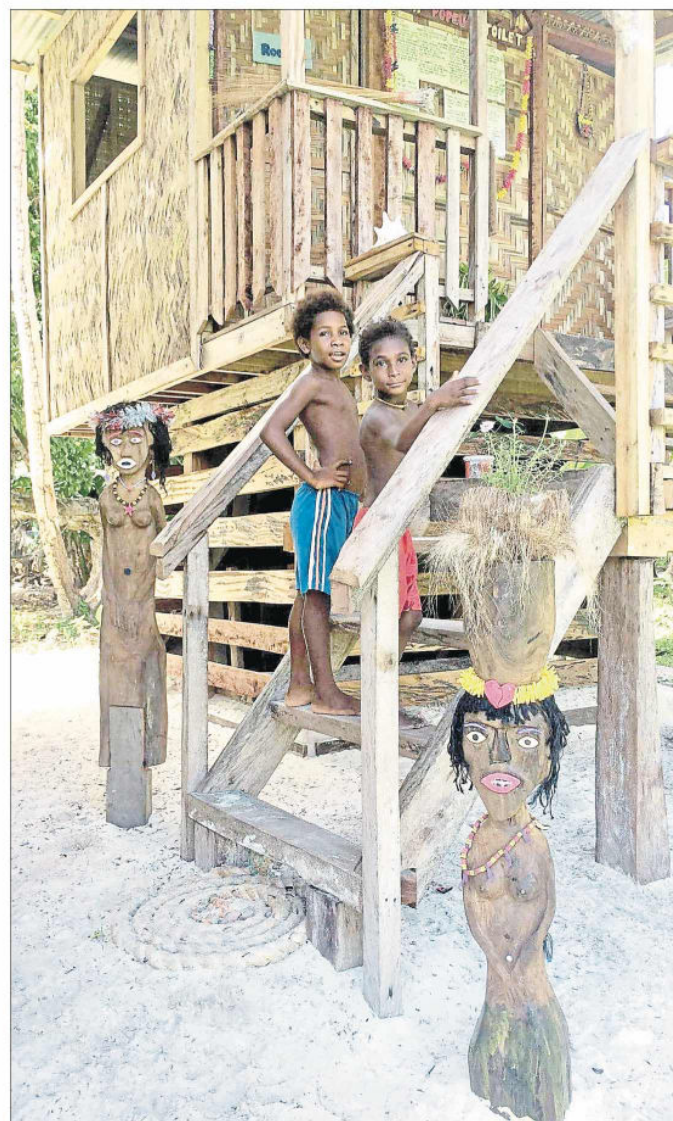
A completed double toilet block at Popeu Village, all bilas-ed!
